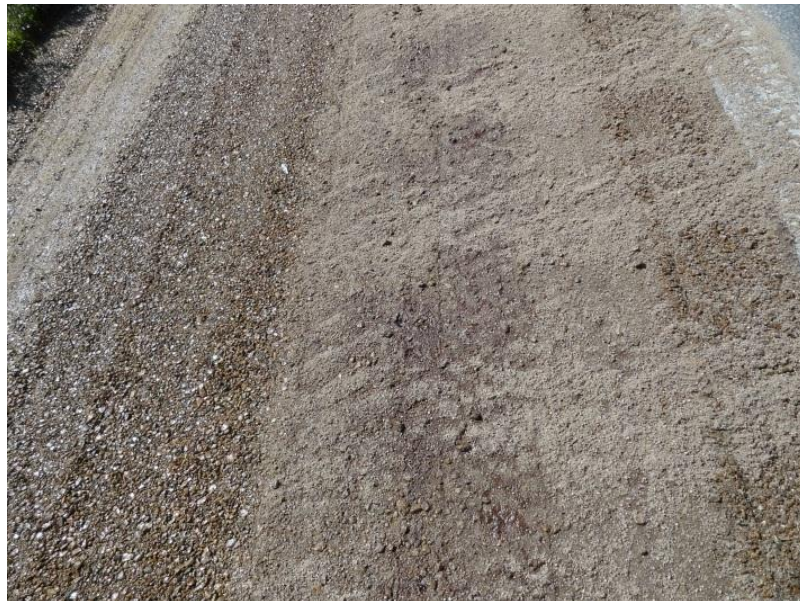
Figure 11. Soapstock and sand applied to recycled asphalt paving materials
