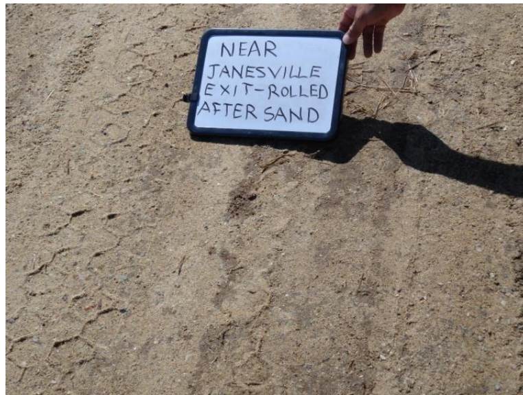
Figure 14. Surface rolled after sand application for the shoulder of US 63 near Denver
