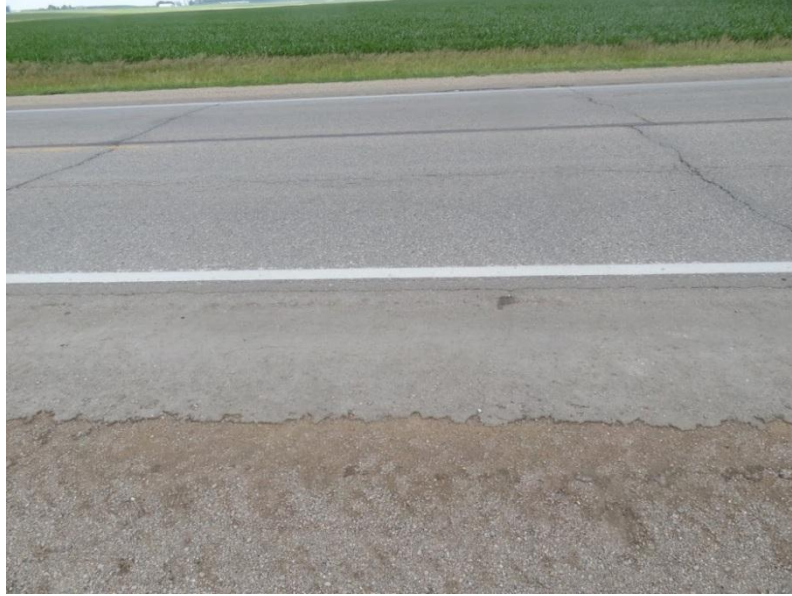
Figure 21. Eastbound shoulder of US 18 near Garner
