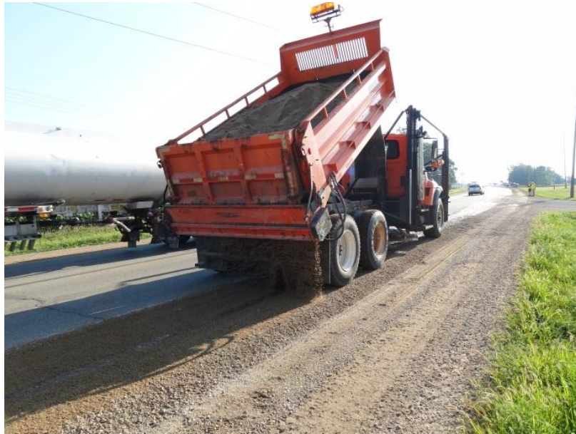
Figure 10. Sand applied on the shoulder of US 18 near Garner
