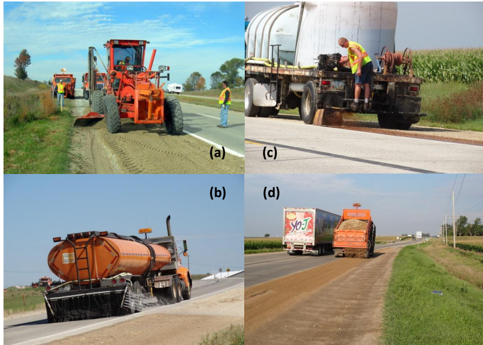
Figure 5. (a) Road grader, (b) water truck, (c) soapstock truck, (d) sand truck
